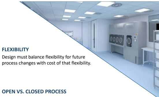
Design should attempt to use closed processes in order to minimize impact to room classifications and flows. Aseptic connections should be utilized to minimize use of isolators for additions and extractions.
