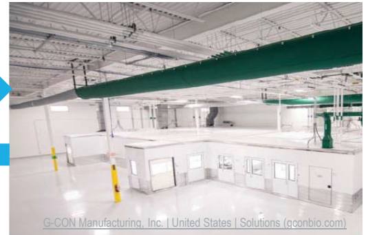
Multiple units in a host structure
